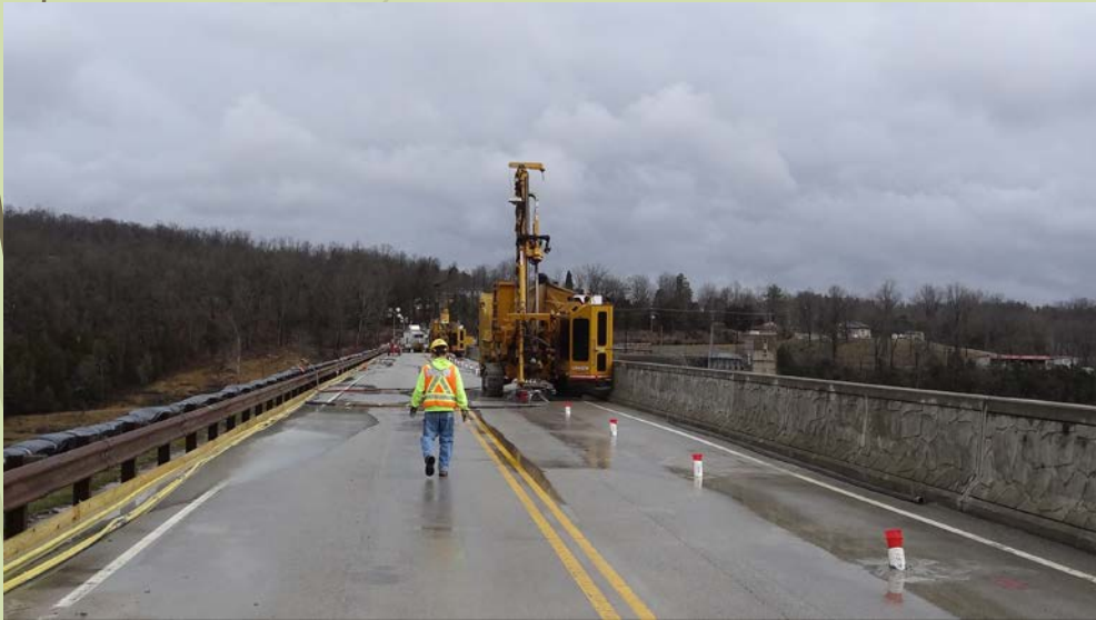
Examples of grouting construction activities at other facilities
