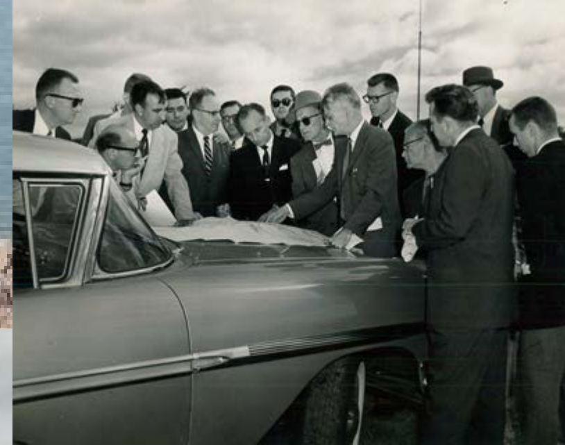
Dike & North Dam during original construction
