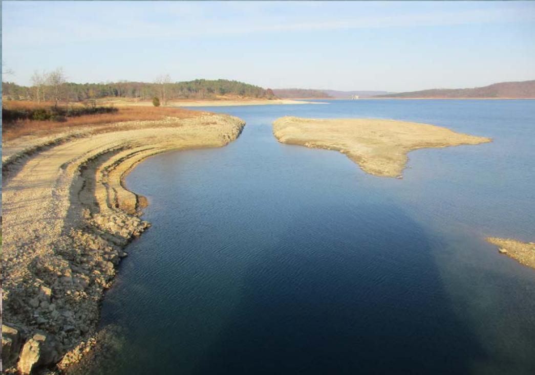
View of the inlet channel from the South Dam Tower
