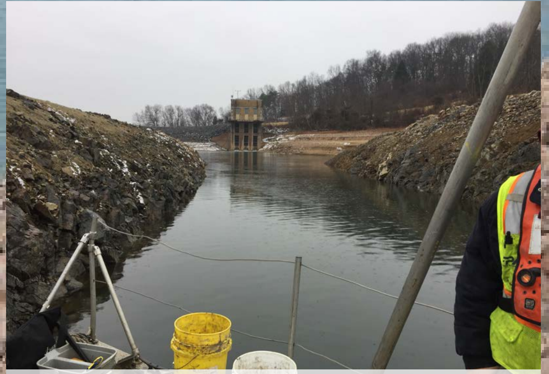
View of the South Dam Tower from the inlet channel
